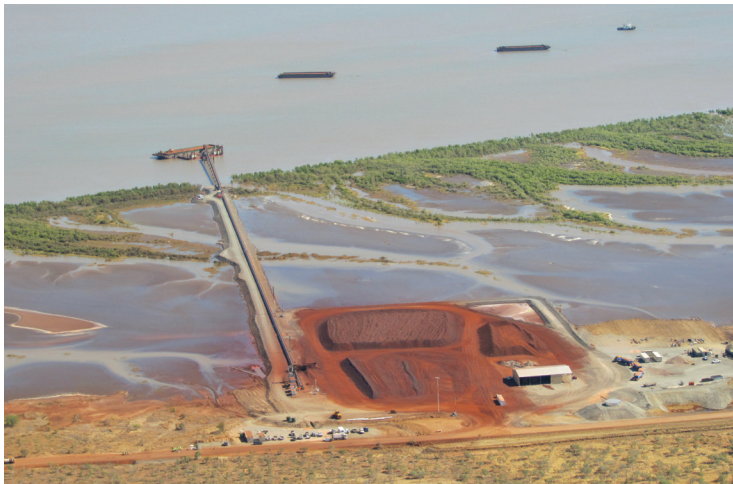
Above: KMG: Aerial photo of site showing overland/overwater conveyor installed over inter-tidal waters (differential settlement a key design parameter)
