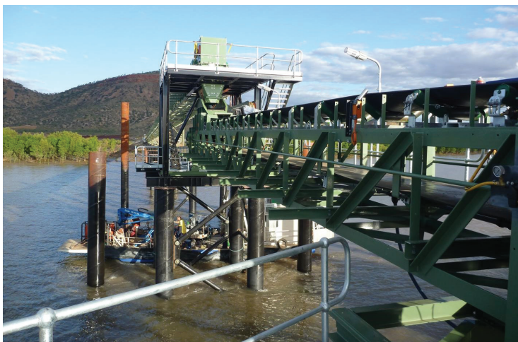
Above: KMG: Aerial photo of site showing overland/overwater conveyor installed over inter-tidal waters (differential settlement a key design parameter)
